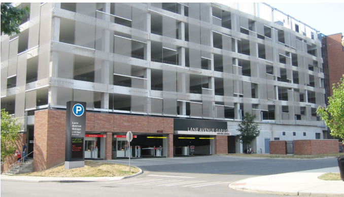
Lane Avenue Garage
