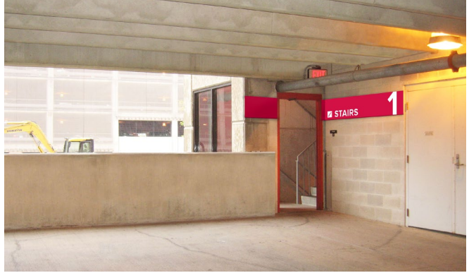
12th Avenue Garage
