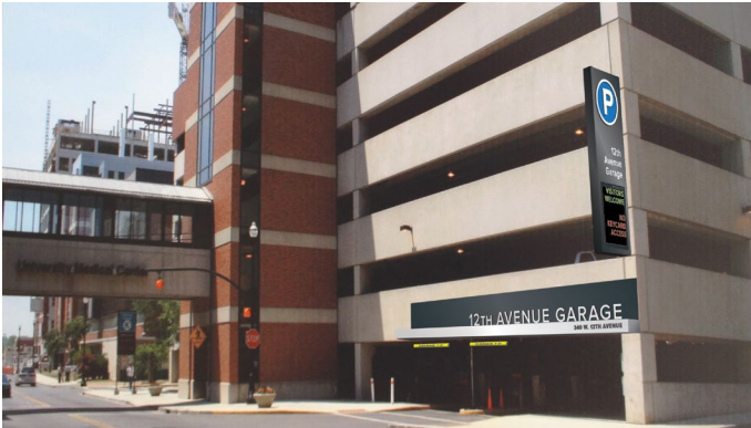
12th Avenue Garage
