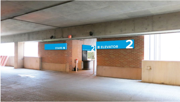
12th Avenue Garage
